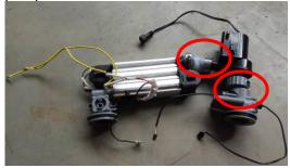
12. Assemble the new PTC heater back into the control box in reverse order. (Video available)
